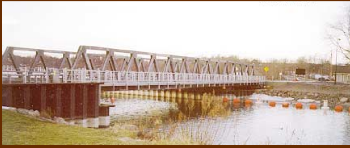
IRONDEQUOIT BAY SEASONAL OUTLET BRIDGE ROCHESTER, NEW YORK MOST DISTINGUISHED PROJECT - 1999
